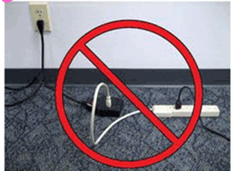
Daisy-chained multi-plug outlets
